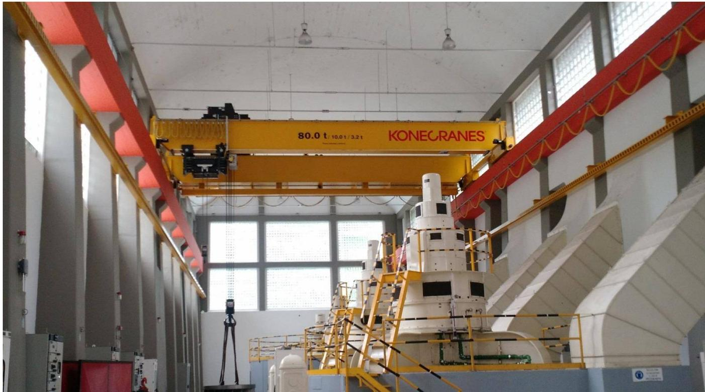
**PUENTE GRÚA 80/10/3,2TON, HIDROELÉCTRICA B. ANCHICAYÁ**
