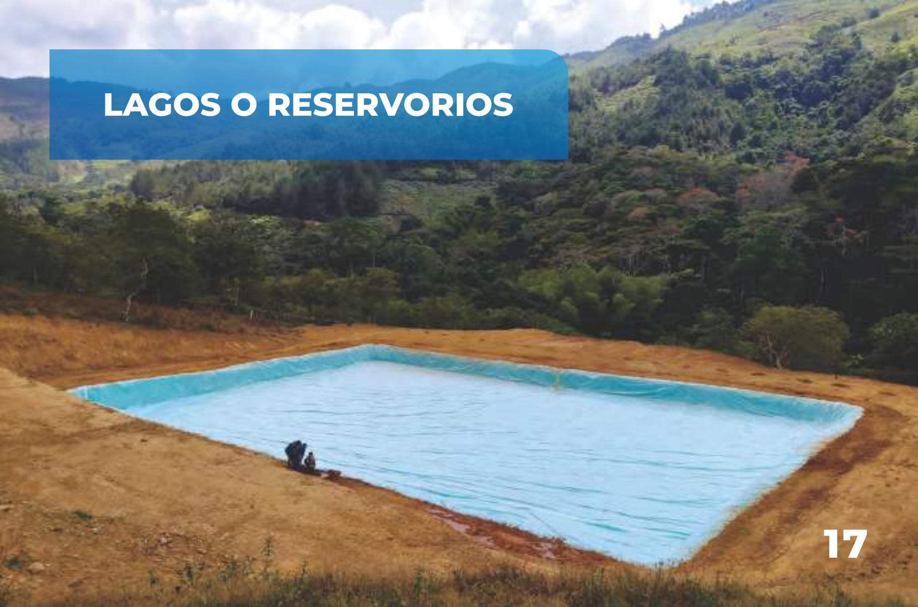
An aerial photograph showing a large, rectangular reservoir constructed in a hilly, forested area. The reservoir is lined with a bright blue geomembrane material, which is visible as a distinct border around the water. The surrounding terrain is a mix of brownish soil and green vegetation. In the background, there are rolling hills covered in dense forest under a cloudy sky. Two small figures are visible near the bottom left corner of the reservoir, providing a sense of scale.
